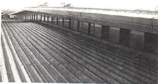
Figure 4. Window type (sliding window) gravity ventilator installed on the roof of a metal working shop
