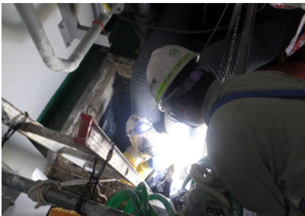
Figure 1. Field photo of dredging work in chemical(liquid lime) storage tank
